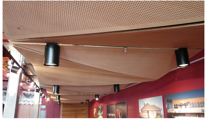
Pre-drilled panels with fabric panels on the backside are an effective.
