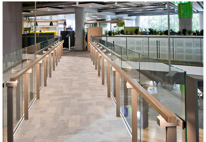
Carpets can be a great way to control impact noises like footfall in high traffic zones.
